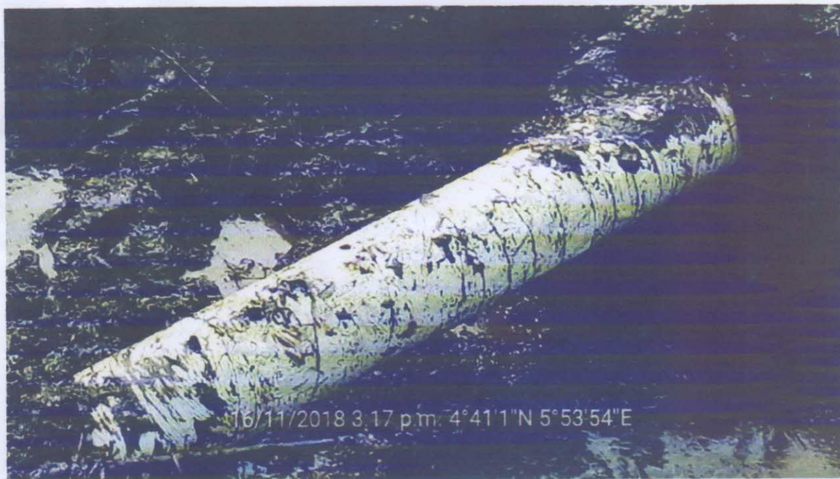
LEAK POINT AFTER REPAIR
